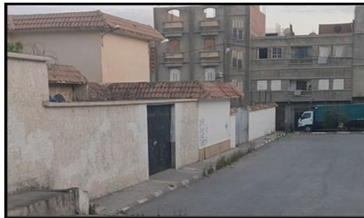
Figure 05: The situation at the educational principal entrance, the absence of architectural installation, and the barbed wire installed directly above the gate
