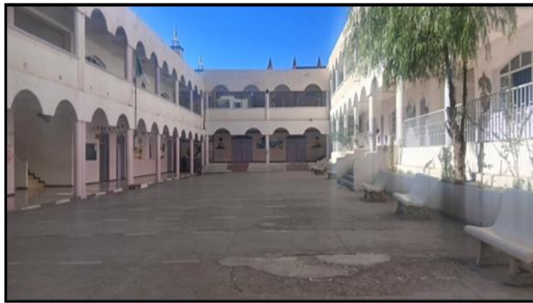
Figure 08: The Central Longitudinal Courtyard in Oortal Bachir Middle school
